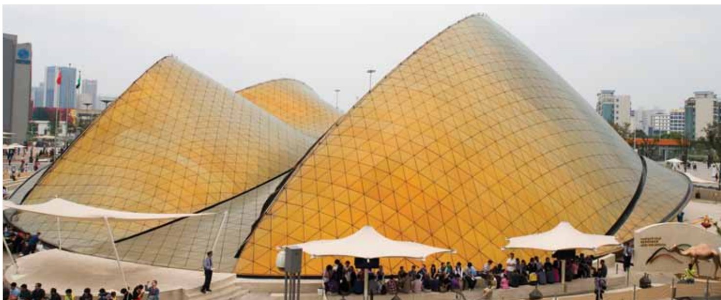
United Arab Emirates Pavilion; view from elevated walkway | 2010 | Image and original data provided by ART on FILE, www.artonfile.com
