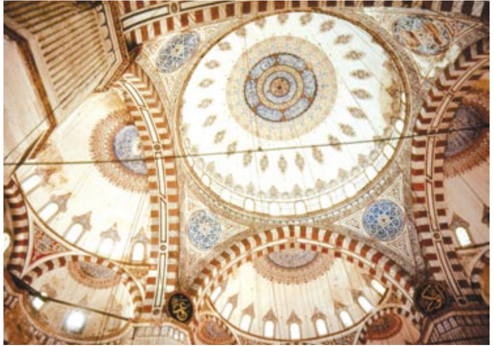
Sinan, architect (1489 - 1588) Mosque of Shehzade Mehmed, Ottoman, ca. 1548 View to the dome and four semidomes, Istanbul, Turkey Image: Walter B. Denny
